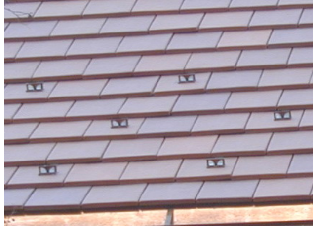
Typical Gough SnoGuard™ for interlocking Ludowici "book" type tiles.
